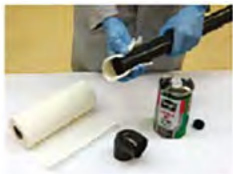
Cleaning the pipe and the socket
