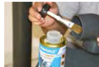
Applying the adhesive
